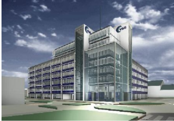
Figure 1 The new ČEZ headquarters in Prague
